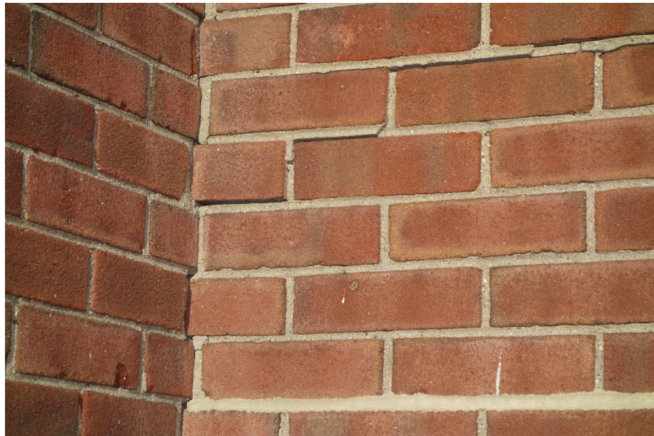
Deteriorated steel lintels, brick ties & mortar joints with brick displacement and cracking
